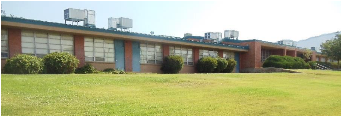
Figure 42. Eubank Elementary (Hesselden, 1956), Linear classroom wing, south elevation.
