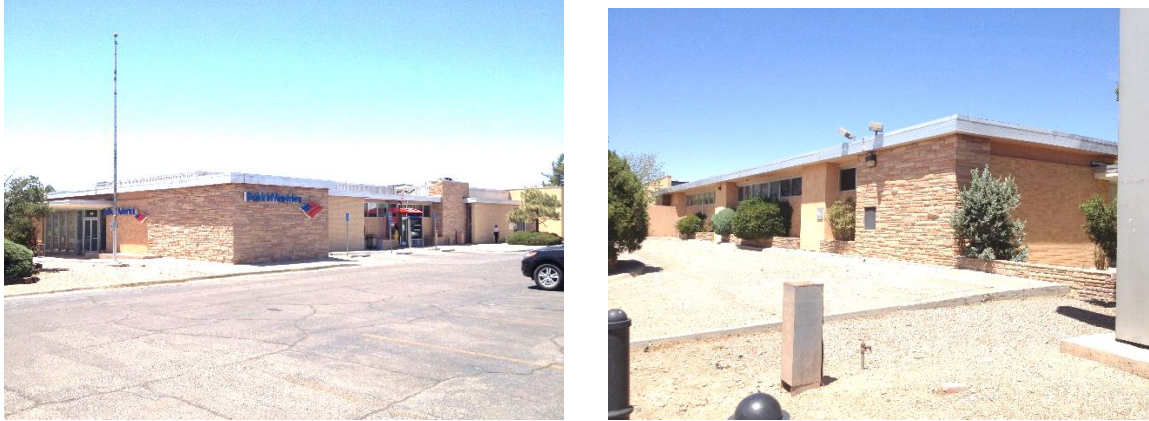
Figure 17. (left) Bank of America branch, south and east elevation. (right) West elevation.
