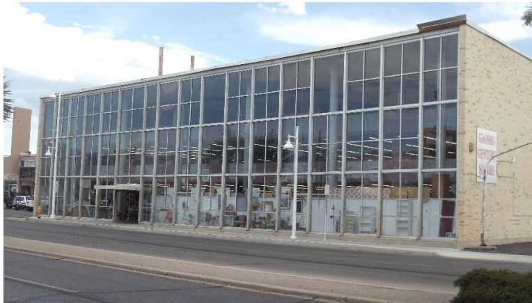
Figure 27. Former White’s Department Store, North elevation.
