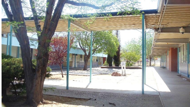
Figure 43. Collette Park Elementary (Stanley and Wright, 1961). Detail of classroom courtyard, overhanging rooflines, and canopies covering walkways between buildings.
