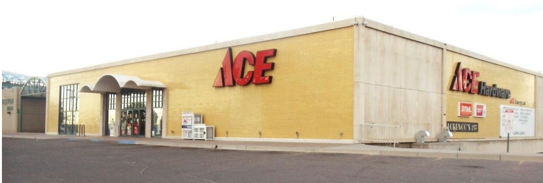
Figure 13. Ace Hardware building, the former Kistler-Collister department store building, West and South elevations.
