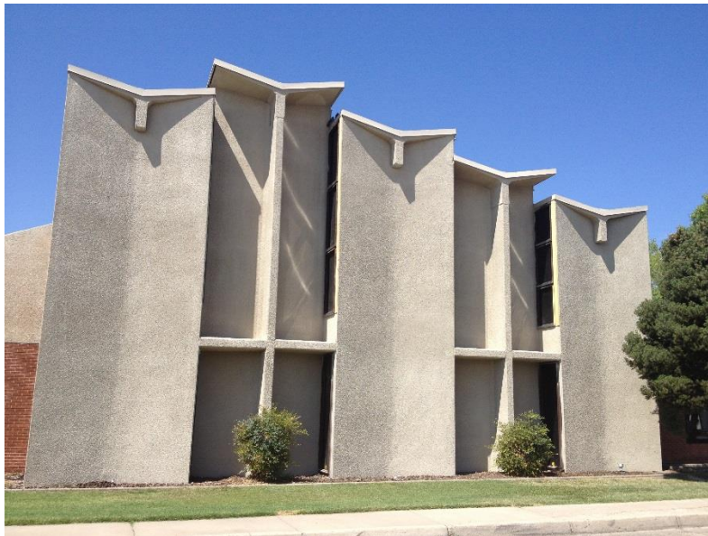
Figure 58. St. Timothy's Lutheran Church, 1968 sanctuary at East elevation.
