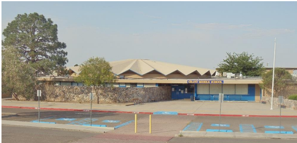
Figure 53. Grant Jr. High (Middle School), front entryway at the North elevation.
