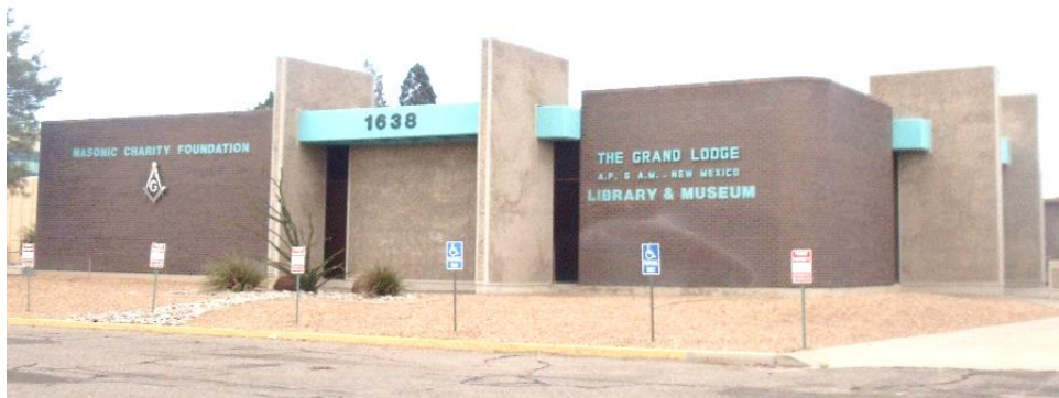
Figure 61. Masonic Grand Lodge, West elevation.
