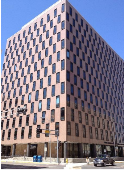
Figure 36. Dennis Chavez Federal Building, East and North elevations.
