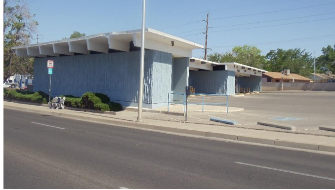
Figure 19. Former ANB Motor Bank, South and East elevations.
