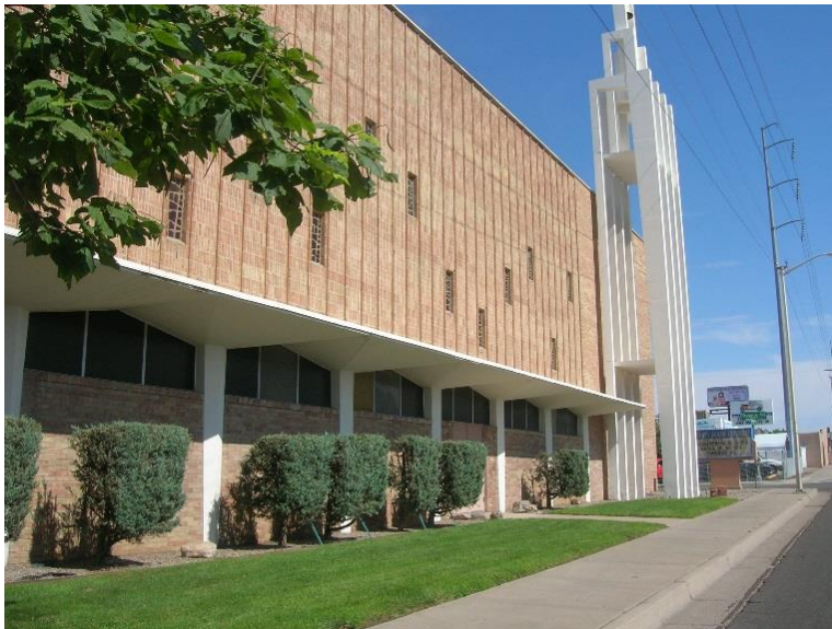
Figure 55. Former Hoffmantown Church, East elevation.
