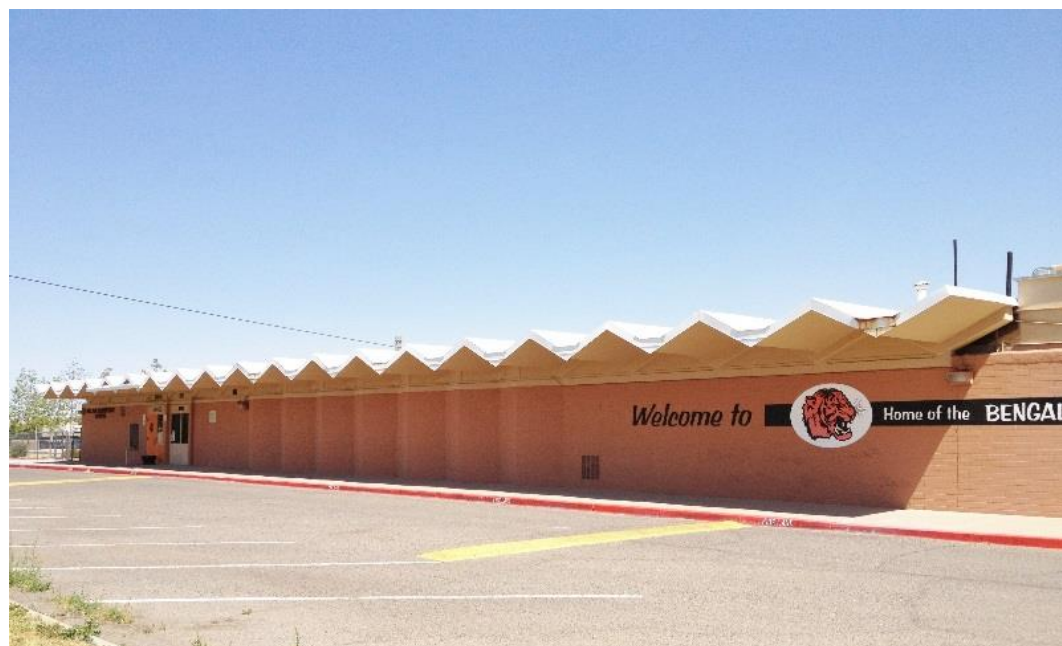
Figure 46. Bel-Air Elementary addition (Flatow, 1960), South elevation showing folded roof plates.
