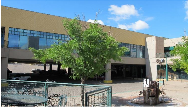
Figure 15. Ace Hardware building. North elevation showing new wall and addition (original wall still intact inside the structure). Note lighter-colored two-story addition at the right side of the photo.
