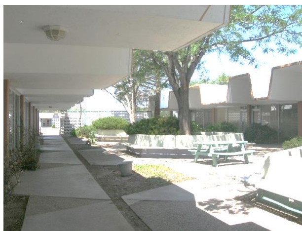
Figure 9. Interior patio at the 6001 building.
