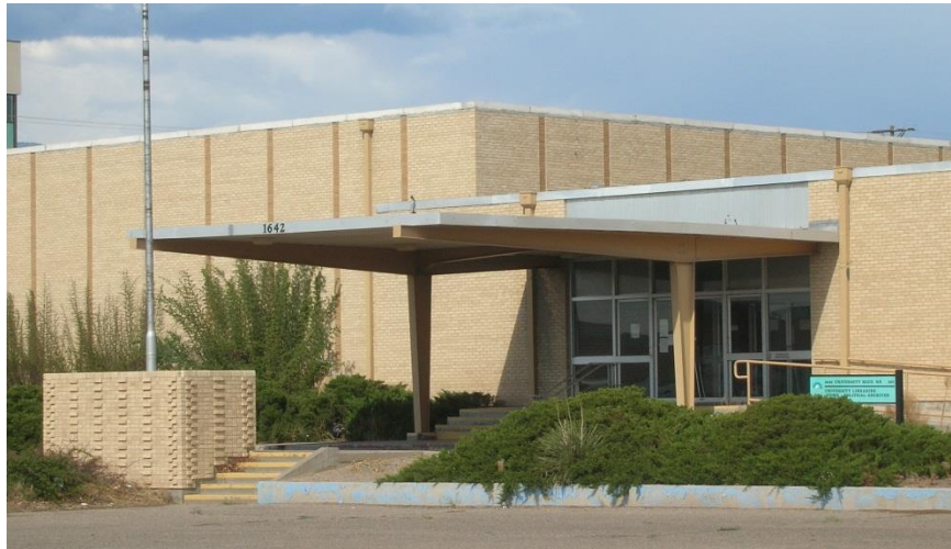
Figure 63. Detail of former Elk's Club front entry canopy.
