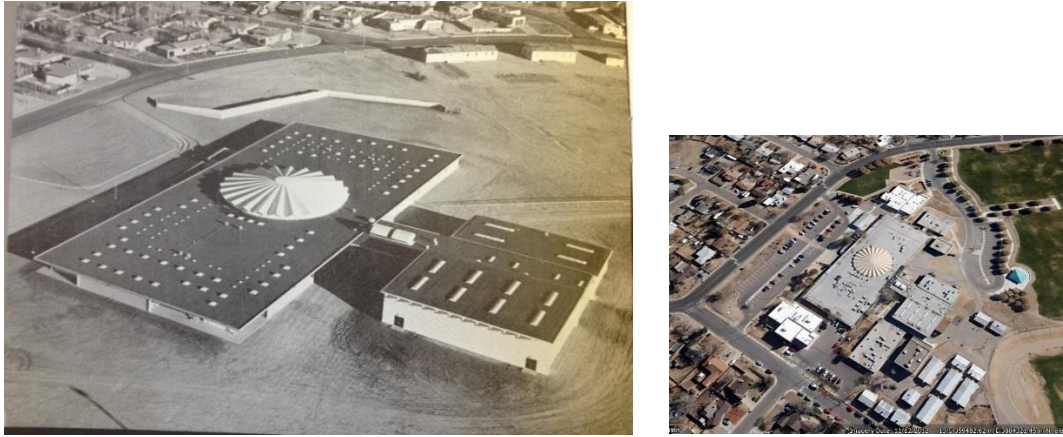
Figure 52. (left) Grant Jr. High (Flatow 1961), aerial view of original buildings, photo taken just prior to opening. Note similarities with Acoma Elementary (Fig. 46). Photo from Albuquerque Progress (1962) (right) Aerial view of Grant Middle School, 2012, note additional buildings since opening. Google Earth image 2012.
