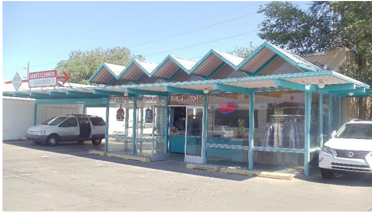
Figure 69. Former One Hour Cleaners (now Arnie's Cleaners and Laundry) located at 8217 Menaul Blvd. NE, South elevation.
