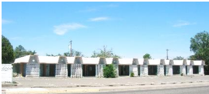
Figure 6. Marble Office Complex. 5905 building, East elevation. The building faces Cardenas St.
