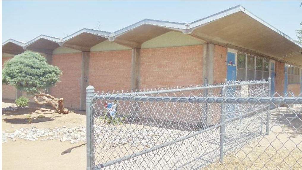
Figure 45. Mitchell Elementary (Ellison, 1962), south elevation showing pre-cast concrete folded roof plates.
