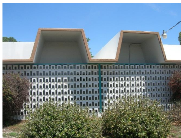
Figure 10. Detail of 5905 building (East elevation) showing pre-cast concrete roof and screen wall.
