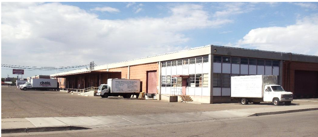
Figure 33. Springer Industrial Complex, 1521C Broadway NE, West and North elevations.
