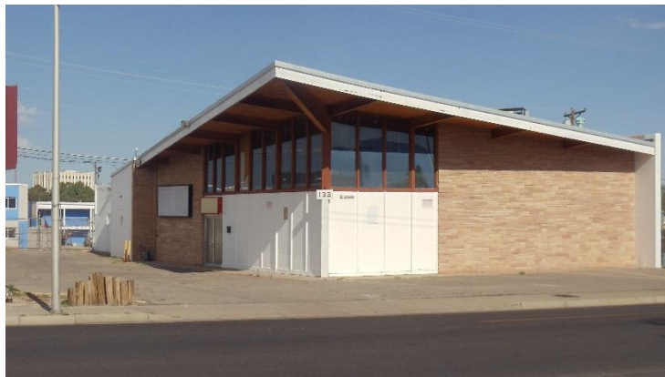
Figure 16. Former Home Builder's Supply building, South and East elevations.
