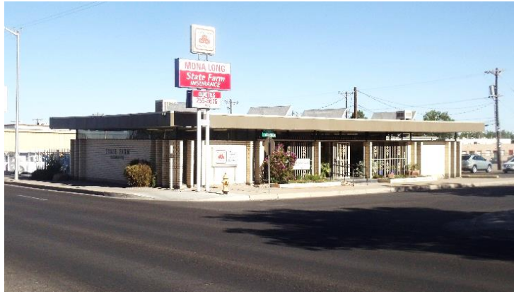
Figure 12: Modernist office building on Lomas, South and East elevations.
