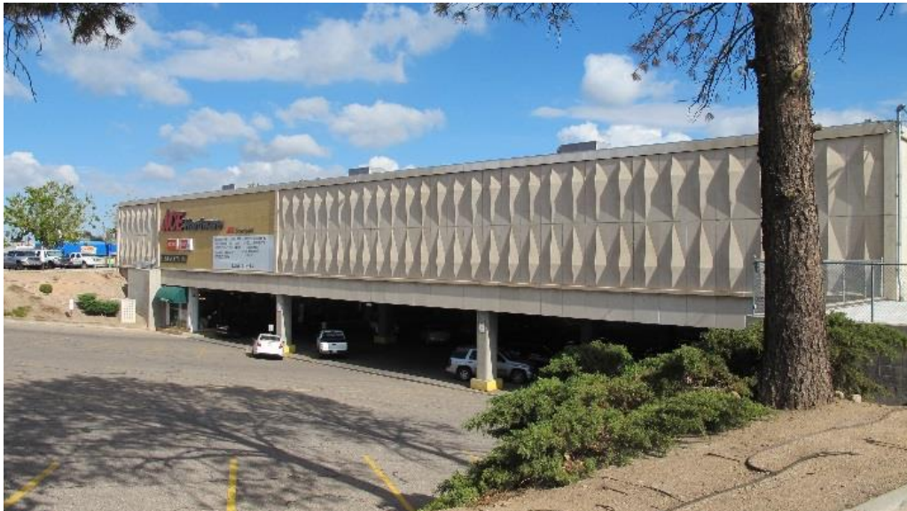
Figure 14. Ace Hardware building. South elevation, showing entrance to lower level parking garage.
