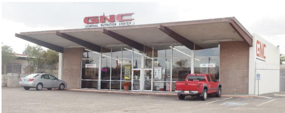
Figure 66. Former Circle K store on San Mateo Blvd. NE, East elevation, reused for a retail business. This building has maintained most of its original features.
