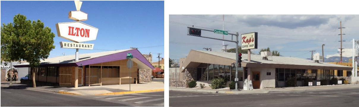
Figure 65. Former Denny's Restaurants on Central Ave. (left) Milton's, South and East elevations. (right) Kap's, West and South elevations.
