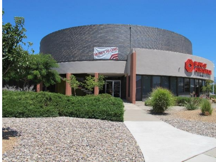
Figure 29. Bank of Albuquerque building, South elevation.
