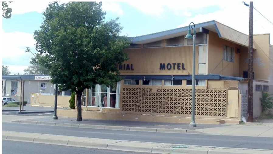
Figure 30. Imperial Inn Motel, distinctive butterfly roof partially obscured, South elevation.
