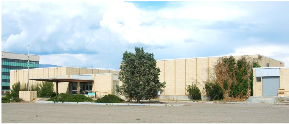
Figure 62. Former Elk's Club, West elevation.
