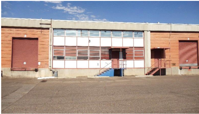
Figure 35. (above) 1605 Broadway NE, mid-bay office at the East elevation.
