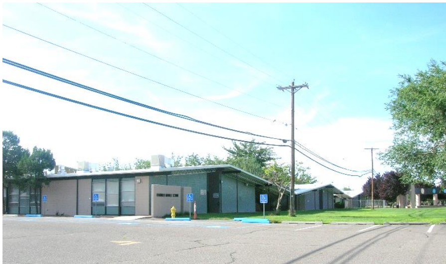
Figure 44. Van Buren Jr. High (Hesselden, 1960), West elevation.
