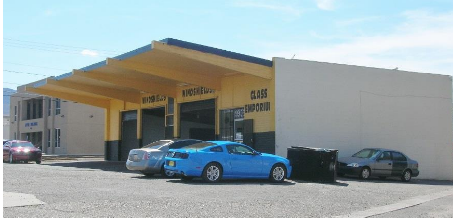
Figure 67. Another former Circle K on Candelaria near Eubank NE, North and West elevations. The roofline remains intact, while the full-height storefront windows have been replaced with garage doors.
