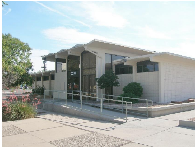
Figure 18. Front entrance to the former Home Savings & Loan building, West and South elevations.
