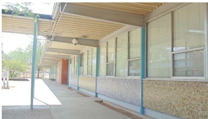
Figure 48. (top) Collette Park Elementary (Stanley and Wright, 1961), detail of mosaics on West elevation. (bottom) Detail of exterior classroom wall showing mosaics below windows. Note also the classic California Plan overhanging roof structure.
